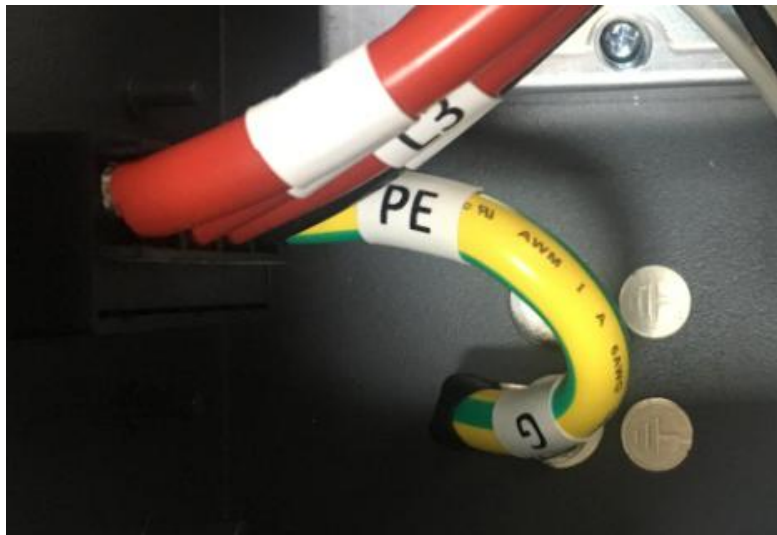
Fig. 12 (HYD 10-20KTL-3PH Ground wire)
